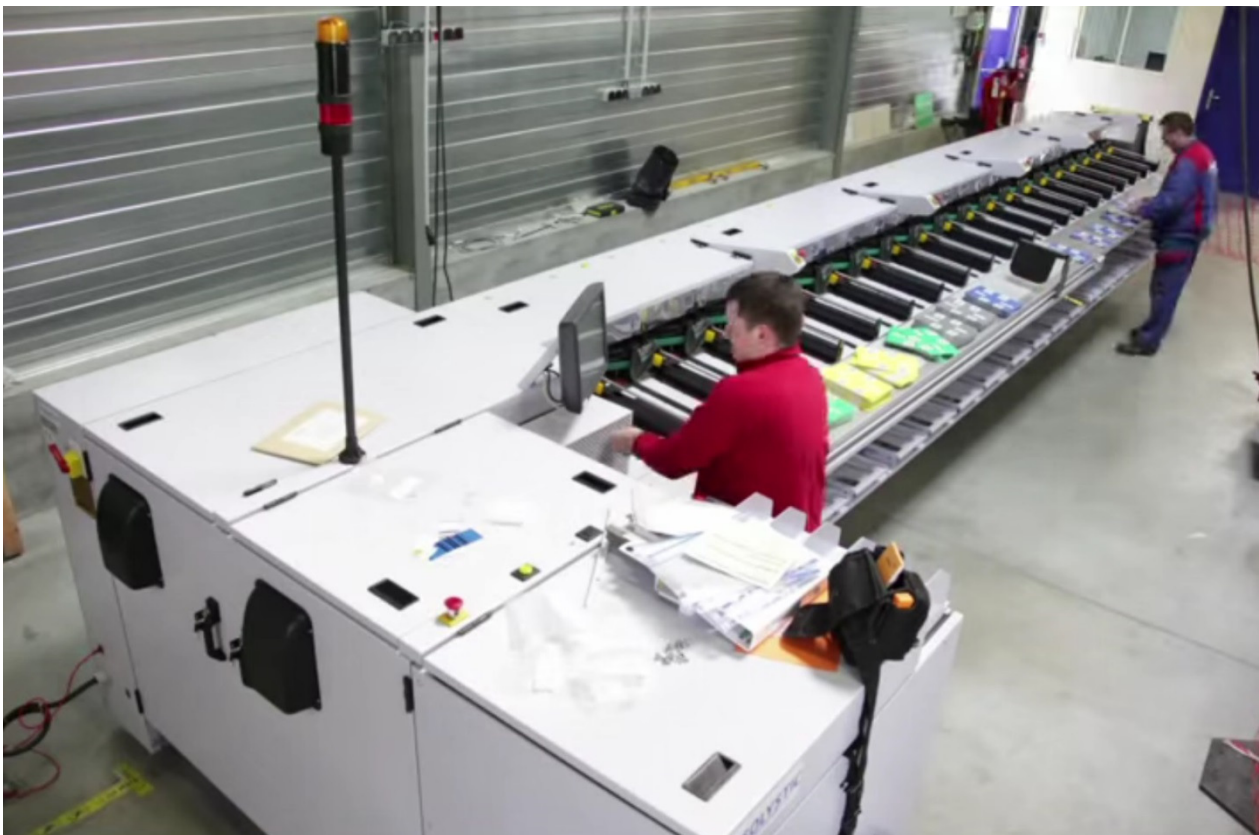
This photograph shows a CSSM being installed at a customer site
